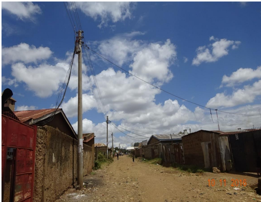
Figure 2: Electricity Connection in some parts of Huruma
