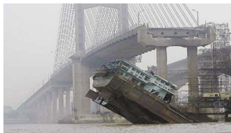
Fig. 1. The highway 325 bridge over the Jiujiang River collapsed due to a ship collision
