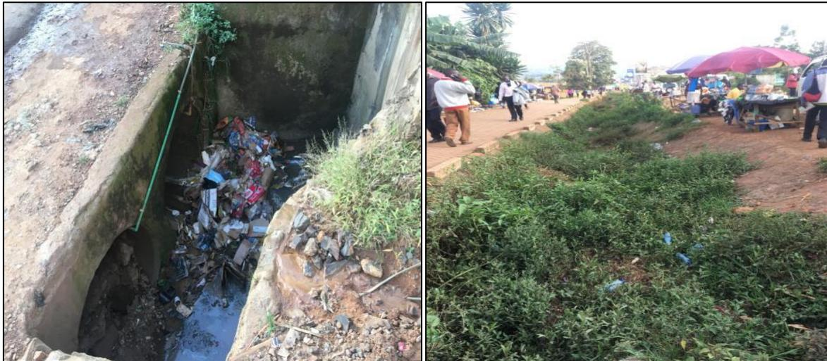
Figure 12: Debris filled and blocked channels (CBD, Mwembe)
